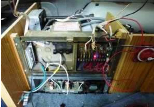
Converter box with wires & circuit breakers removed from 120 VAC electrical panel.
