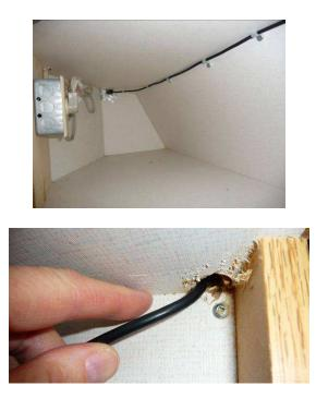
Figure 3 and 4. Camera cable path through upper left side cabinet.
